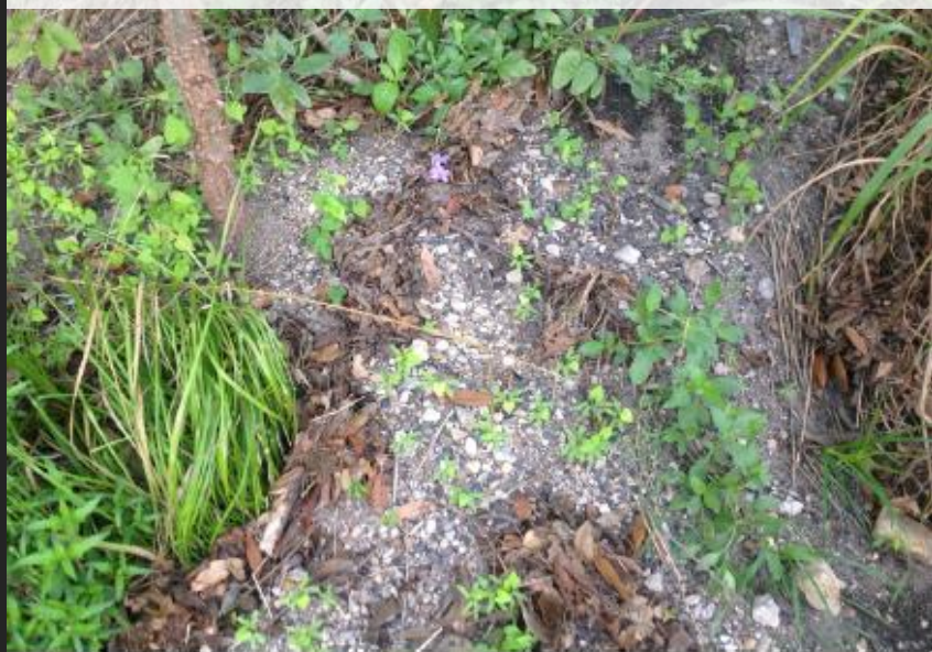
SEDIMENT DEPOSITED IN BASIN
