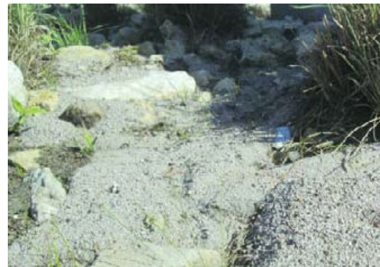
Sediment in Rain Garden
