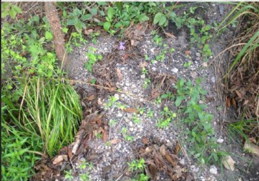
SEDIMENT DEPOSITED IN BASIN
