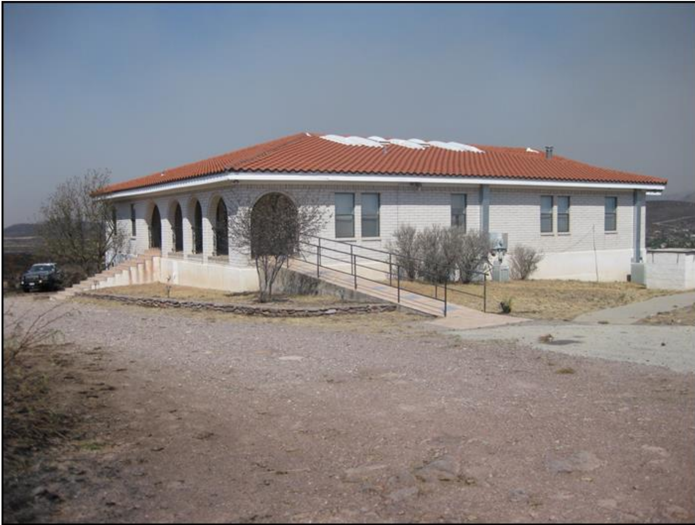
Driveway and yard on East side of home. Facing Delores Mountain Drive.
