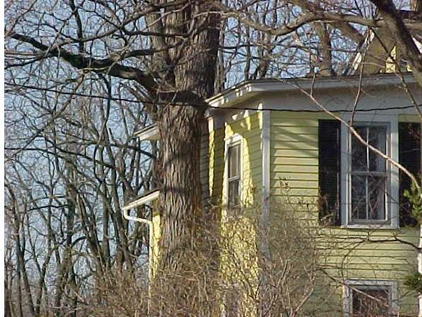
Gunther Home Inspections
