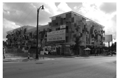
The East Village on 11th Street, once a lot with dilapidated structures, now provides residences above a retail area
