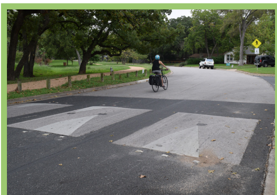
Asphalt Speed Cushion
