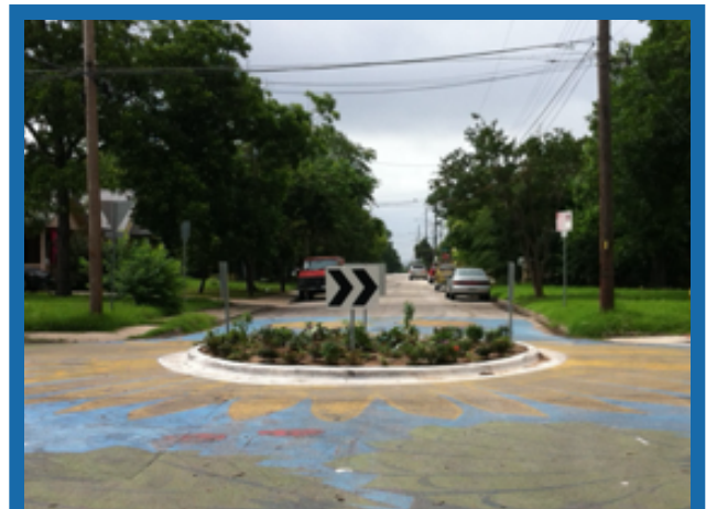
Traffic Circle with Raised Curbs
