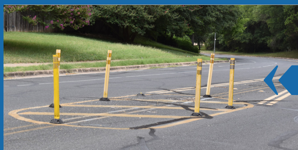
Rapid Build Median using Delineators
