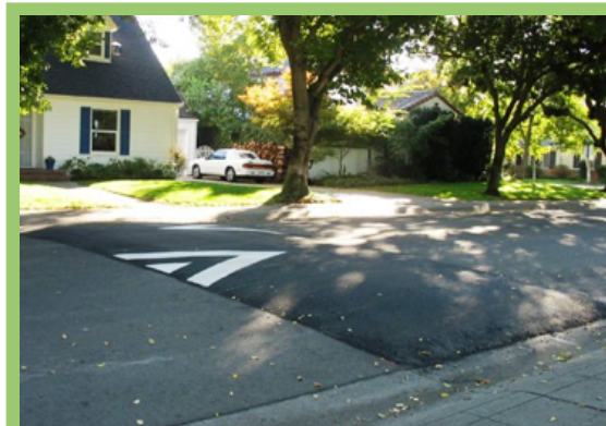
Asphalt Speed Hump
