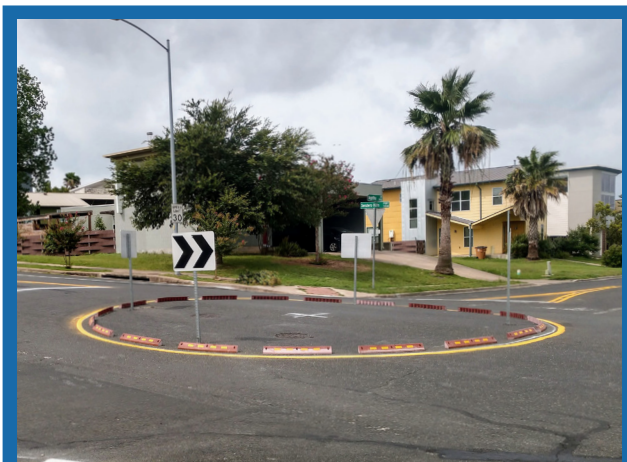
Rapid Build Traffic Circle
