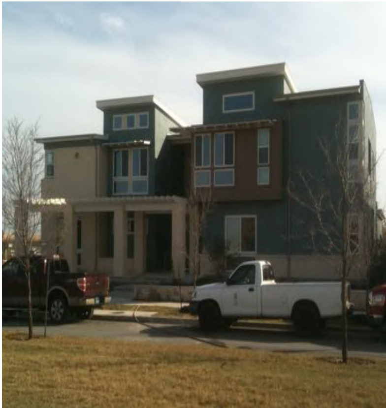
Mueller Fourplex: 7,017 sq ft, 9677 sq ft lot (0.73 FAR) Corridor bonus max: 7170 sq ft (0.74 FAR)
