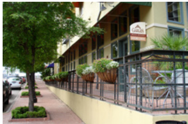
A terrace with outdoor seating that wraps around the building corner.
