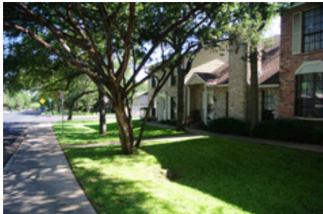
The front yards of these rowhouses form a continuous common yard.
