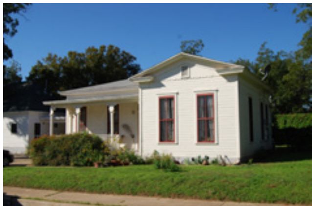
An engaged porch as an attached element leading up to the entrance.
