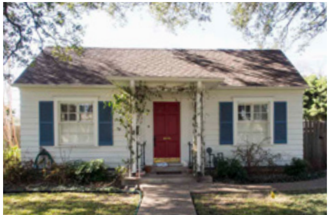
A stoop on a small detached house.
