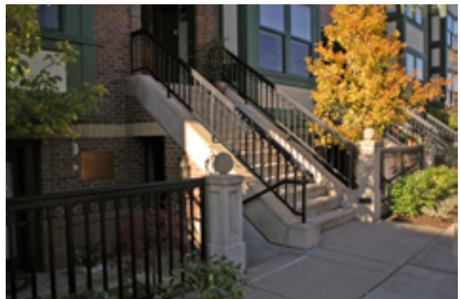
Lightwell frontage for a rowhouse building.
