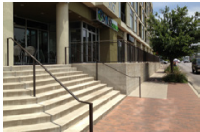
A terrace used to accommodate a change in grade.
