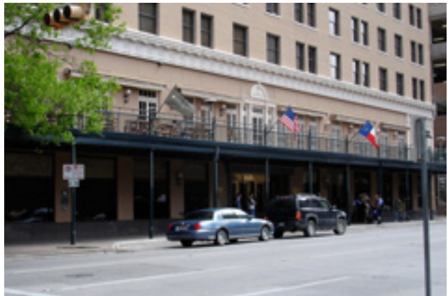
A single-story gallery with second floor access to the spaces on the upper story.
