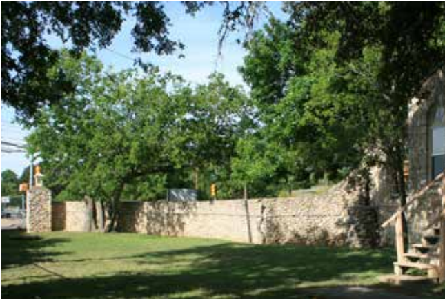
Figure 535. Limestone retaining wall (John Milner Associates)
