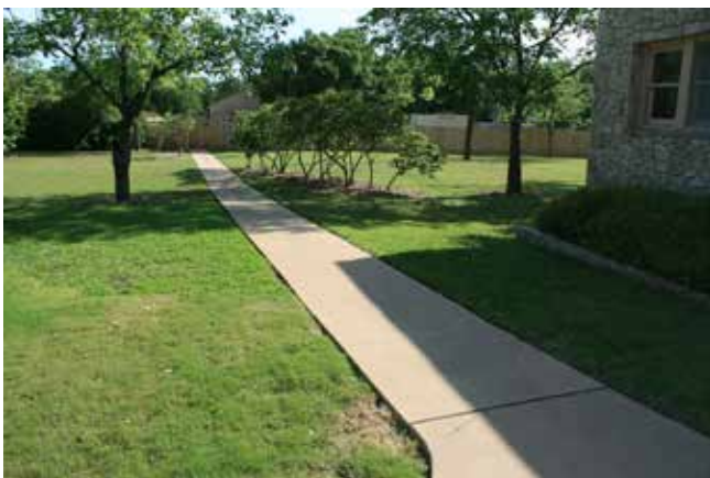
Figure 455. Concrete sidewalk leading from the cemetery office to the maintenance complex (John Milner Associates)
