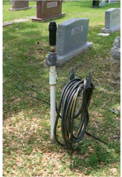
Figure 526. Irrigation riser with attached hose and decorative hose rack (John Milner Associates)
