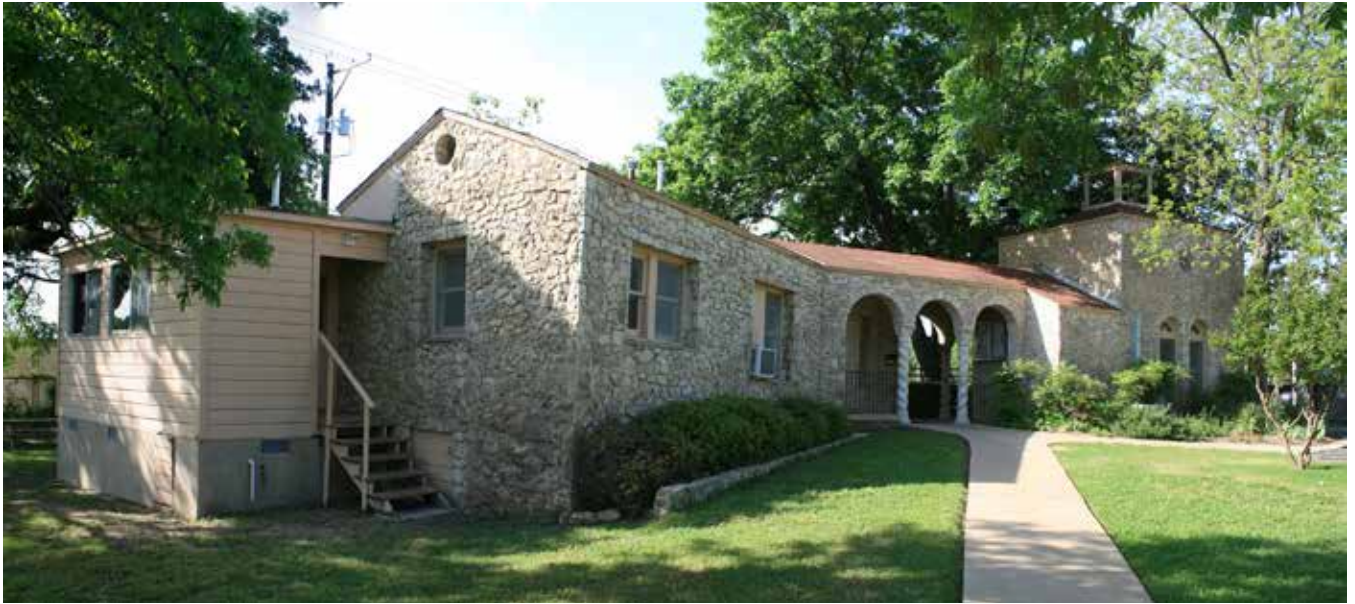
Figure 531. The cemetery manager's office (right) is connected by a breezeway to the larger building that once served as the cemetery caretaker's residence. (John Milner Associates)
