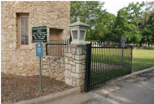
Figure 538. Rock piers support the entrance gate. (John Milner Associates)
