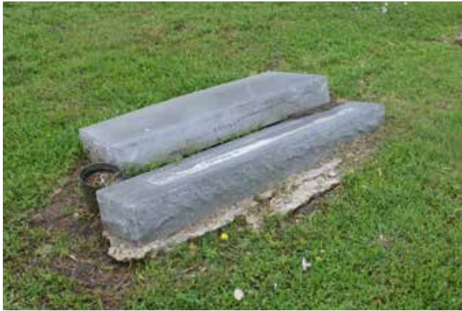
Figure 506. A marker with an exposed concrete foundation (McDoux Preservation)
