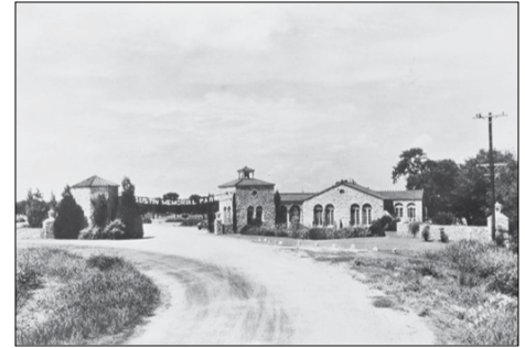
Figure 430. Entrance to Austin Memorial Park Cemetery, undated photograph, showing service tower to the left of the gate and chapel/cottage to the right (Austin History Center)
