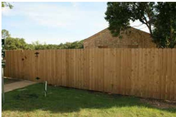
Figure 542. A wood privacy fence surrounds the maintenance area; the pedestrian gate is visible on the left. (John Milner Associates)
