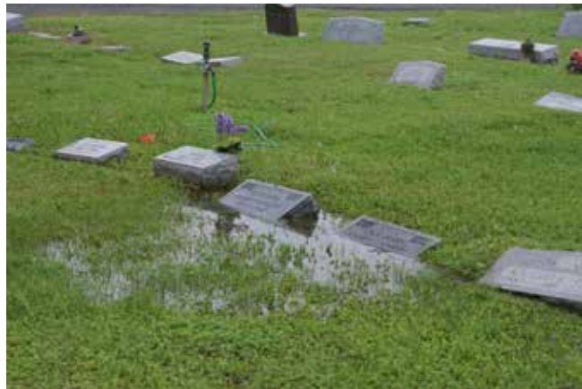
Figure 511. Ponding and subsidence in Section 7 (McDoux Preservation)
