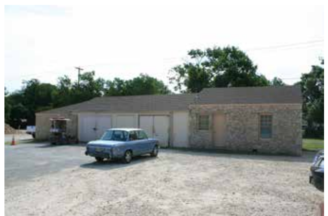
Figure 534. Cemetery maintenance building, formerly the cemetery office (John Milner Associates)
