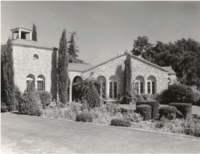
Figure 478. An undated photograph showing the former sunken garden (City of Austin)
