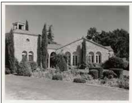
Figure 432. Sunken garden at Austin Memorial Park Cemetery, undated photograph (Historic American Buildings Survey)
